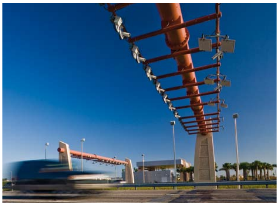
Funded by tolls, MDX has been aggressively upgrading and updating its roads over the past decade
